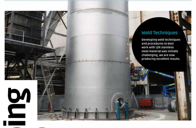
Wulguru Group is constructing a 70m high boiler stack for the Macknade Sugar Mill.
